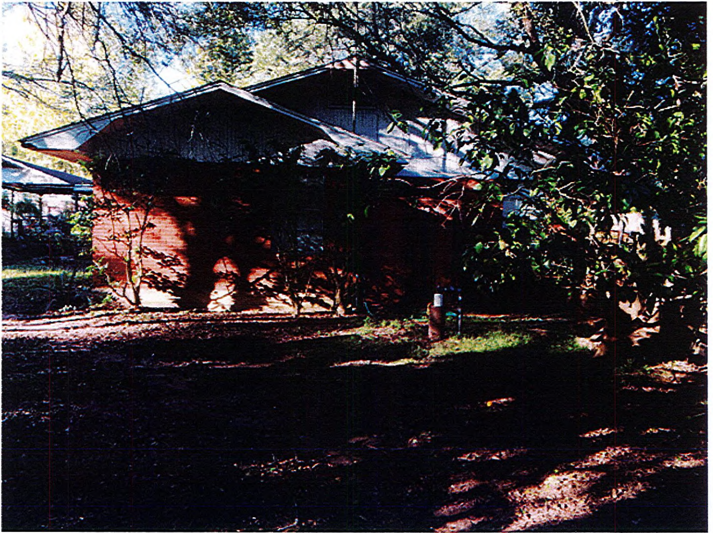
South side of building
