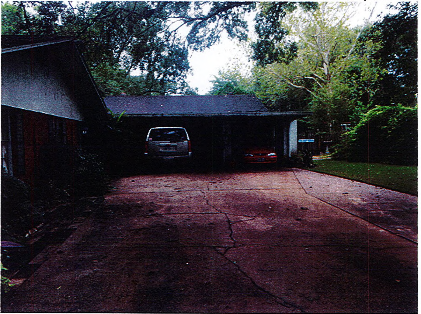
North side of building
