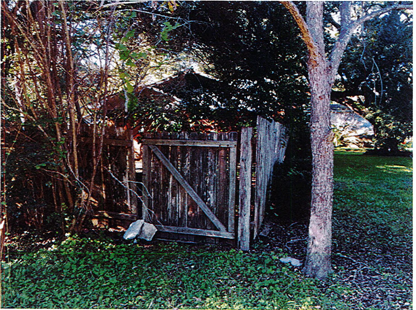
South side fencing – plan is to move/refurbish fencing following city ordinances
