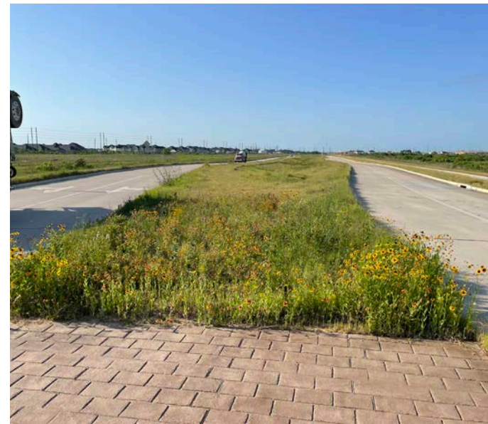
2 MORGANS SPUR DRIVE - S MEDIAN LOOKING SOUTH
