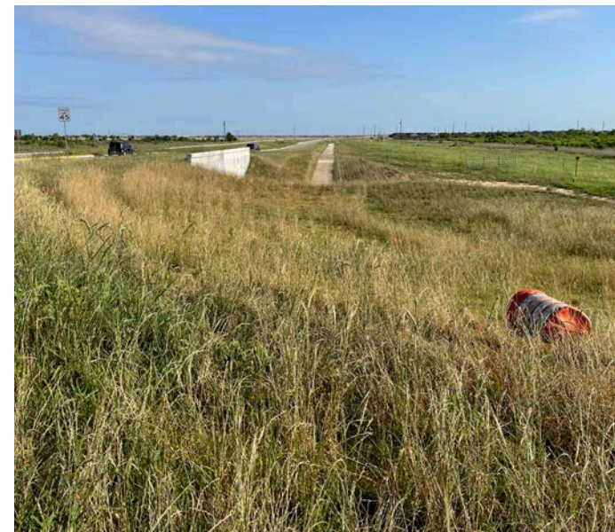
6 TAMARRON PARKWAY - NE CORNER E-W UNDERPASS VISIBLE
