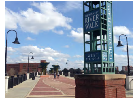
Example of Minor Gateway Signage
