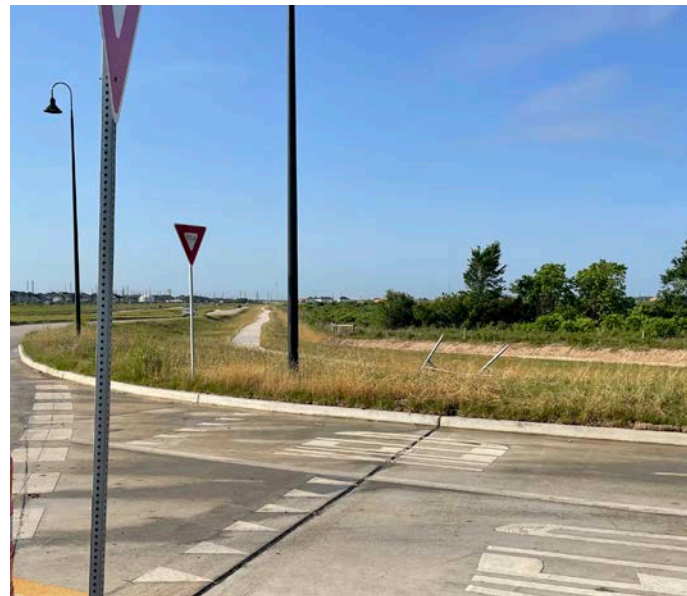
1 MORGANS SPUR DRIVE - SW CORNER LOOKING SOUTH
